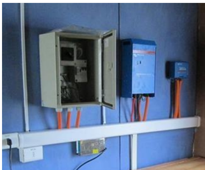
FIGURA 31: INSTALACIÓN INVERSOR OFF GRID EN AYSÉN (B. MUNIZAGA)
